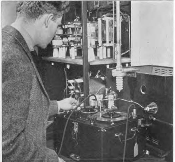
FIGURE 1. Adjusting antenna coupling networks at Radio Station WHDH with the TYPE 916-A Radio-Frequency Bridge.
